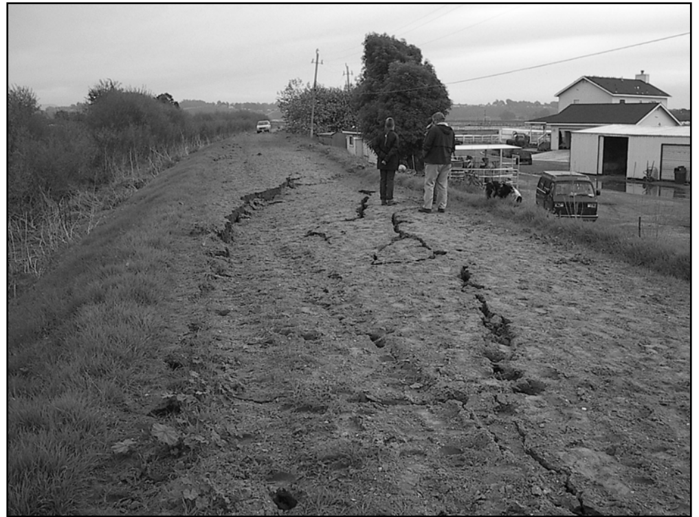
Damaged Levee
